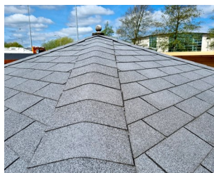
FELT SHINGLE ROOF
