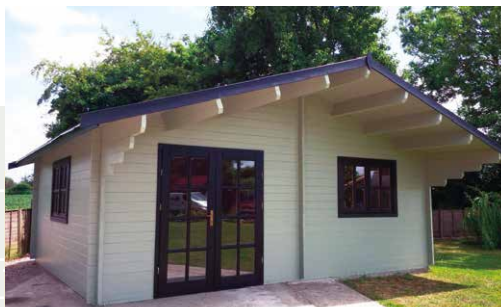
Picture supplied by customer on completion, 2 colour paint finish
