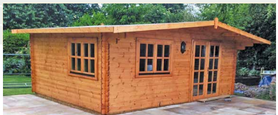
Picture supplied by customer on completion
